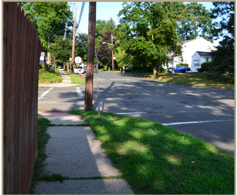
Figure 15. Missing curb cuts and ramps
