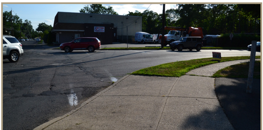
Figure 37. Looking southwest across Madison Avenue at South Avenue
