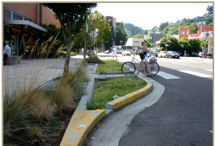
Figure 9. Green infrastructure used to narrow the roadway and provide a shorter crossing distance for pedestrians.
