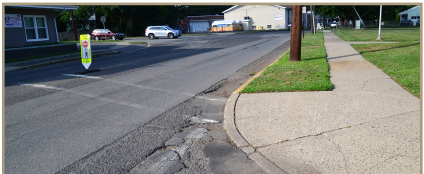
Figure 33. Looking north across South Avenue at South Madison Avenue
